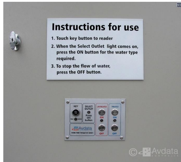
Typical Control Panel
